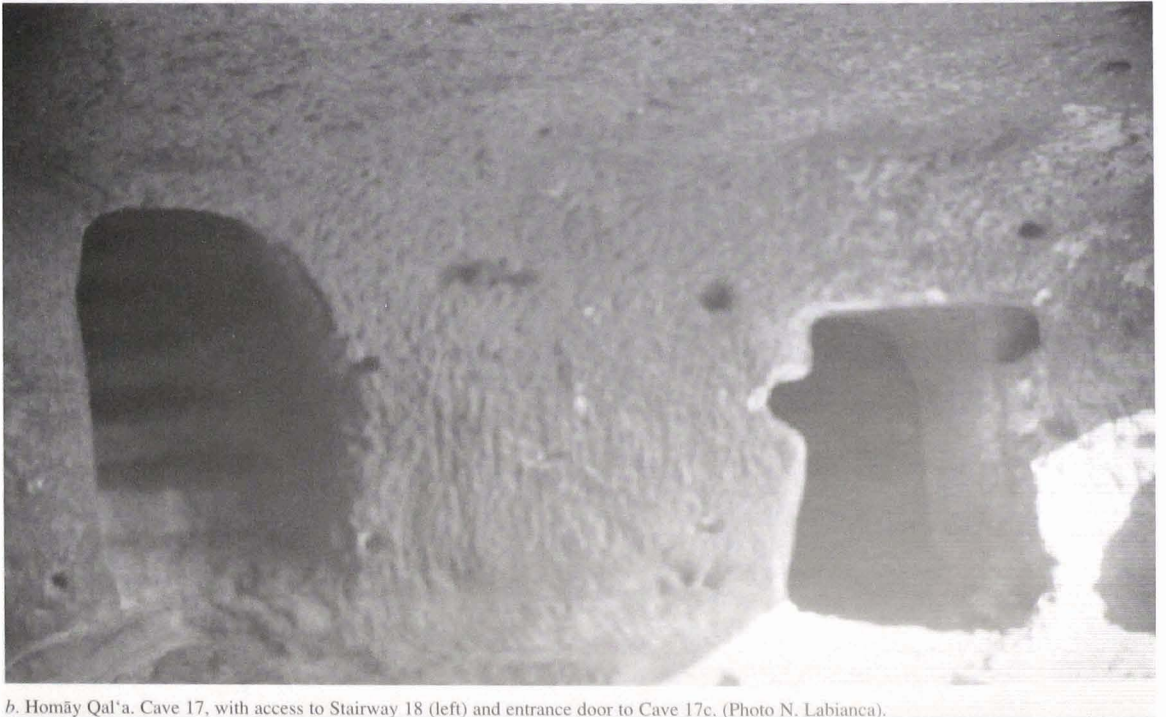
b. Homāy Qal'a. Cave 17, with access to Stairway 18 (left) and entrance door to Cave 17c. (Photo N. Labianca).
